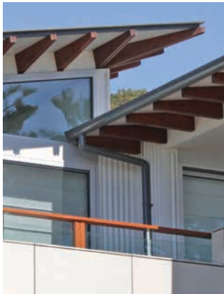
Detailing under eaves and circular downpipes
