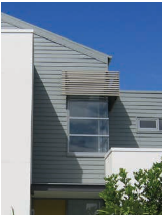
Effective sun shading devices
