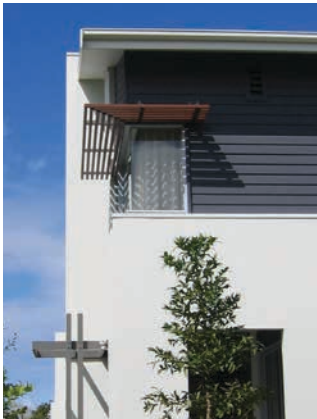
Effective sun shading devices
